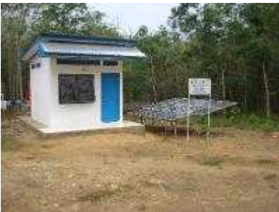
Place of installation
